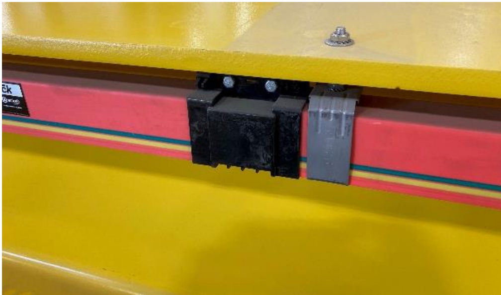
2.7.3 Plastic Splice Cover Connecting Rails Together
